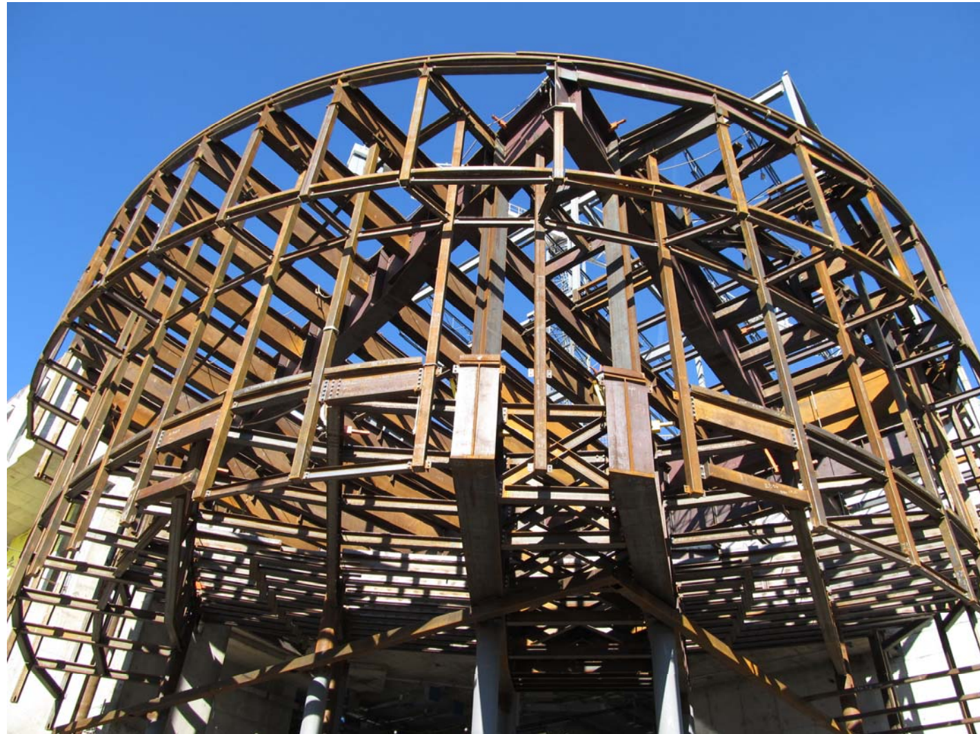
Drum—Support Framing
